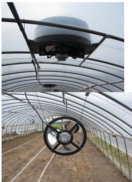
Figure 1: Forced-ventilation (top) and air circulation treatment (bottom) in the plastic house
